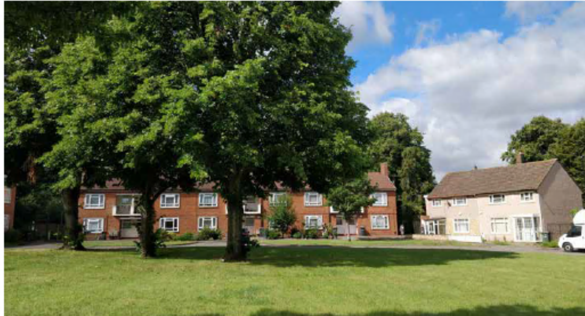
8. View South West to Phoenix bedsits with line of Category A trees.
