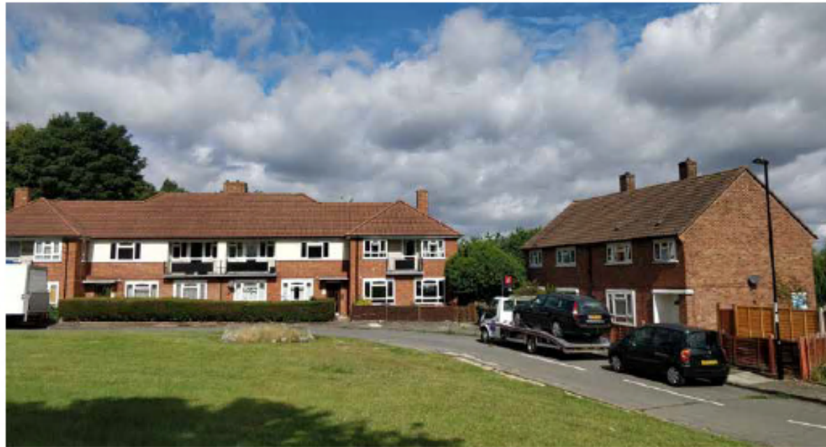
6. View North West to vacant 3-10 Chingley Close, to be cleared.
